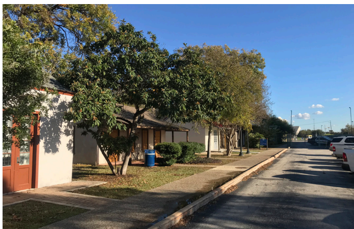
Fig. B.4-1: Existing Historic Structure Along E. Nueva Street
