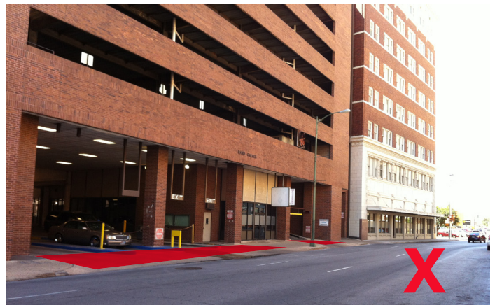
Fig. C.6-4: Unacceptable Street Side Service Zone
