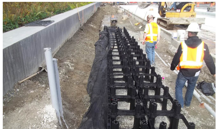
Fig. C.2-3: Silva Cell Installation
