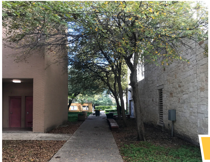
Fig. C.4-2: Existing Fire Department Access to the Henry B. Gonzalez Convention Center from
