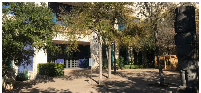
Fig. A.4-7: Existing Henry B. Gonzalez Convention Center Southwest Entry
