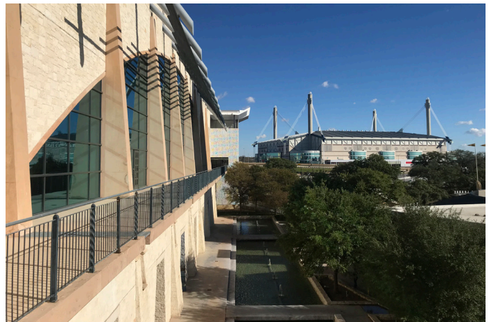
Fig. A.4-5: Existing Henry B. Gonzalez Convention Center South
